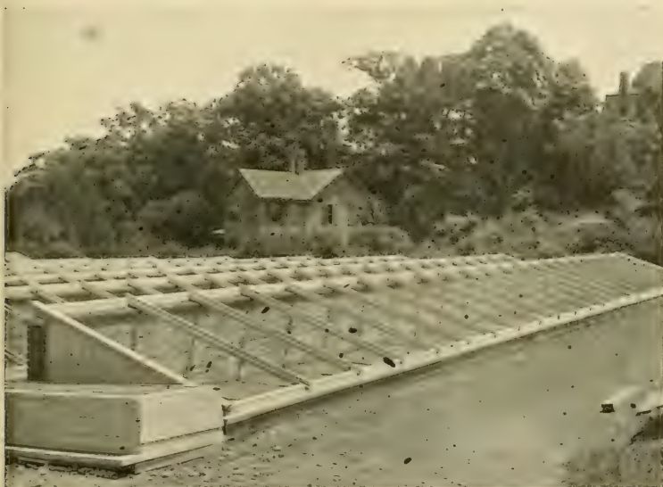
Coldframes of brick and iron
